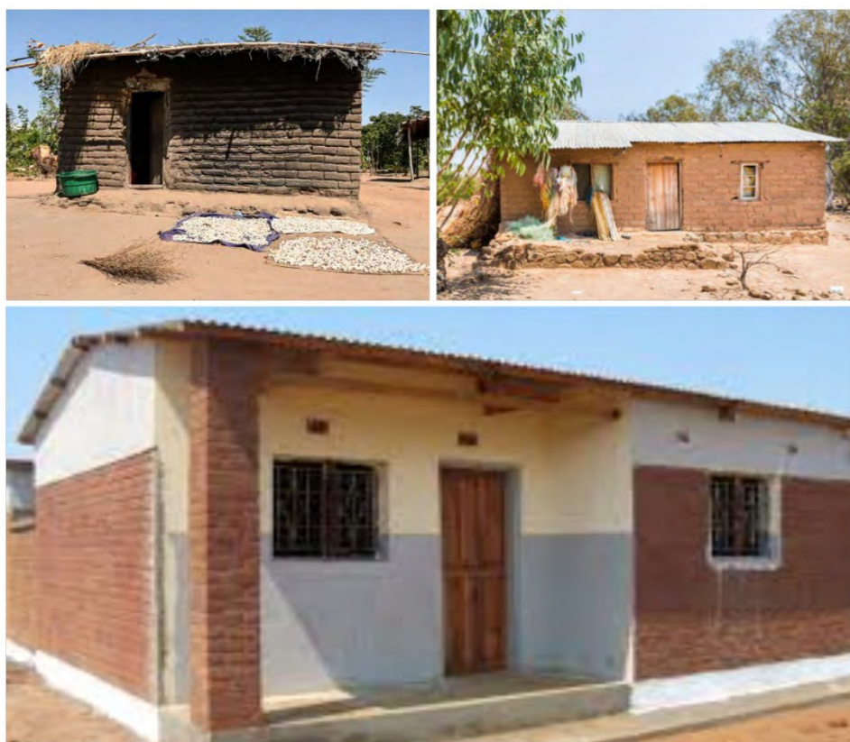
Figure 3-1: From top left; Traditional, semi-permanent, and permanent house
